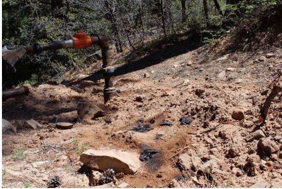
Figures 5 and 6 - Spilled oil and poorly maintained piping observed in 2018 at Navajo 24.
